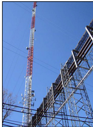
PARTIAL VIEW OF ANTENNA AND COAXIAL RF FEED.
