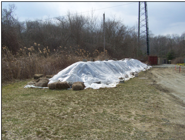
MINI-ALPS - WHAT'S LEFT FROM EXCAVATING THE MATERIAL FROM THE OIL SPILL.
