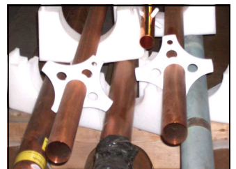
COAX CENTER CONDUCTORS.
