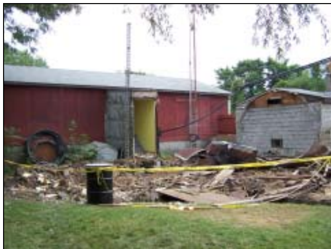
THE QUONSET HUT IS REMOVED
