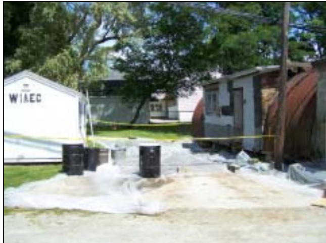
COVERED SITE - FIRST DAY
