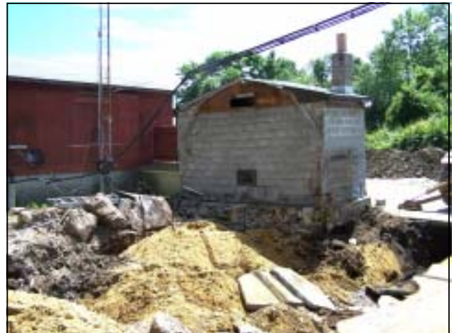
FURNACE BUILDING, PARTIAL BACK FILL
