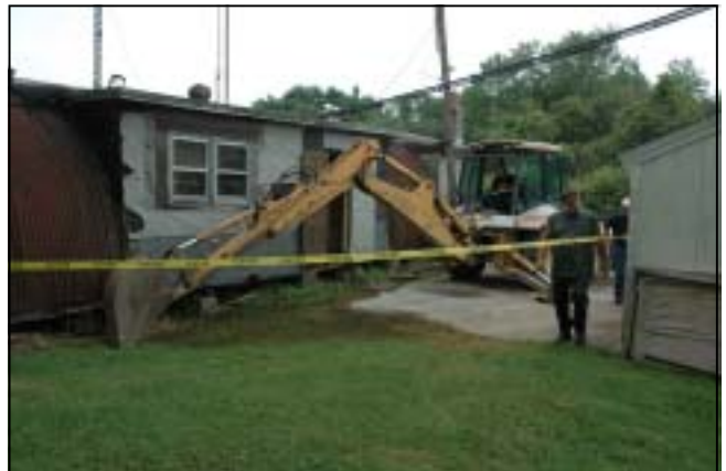
DIGGING THE FIRST TRENCH
